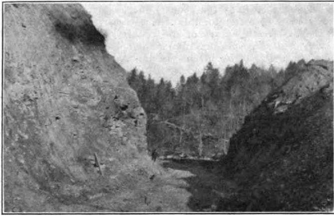
Heavy Cut at Mile Post 83; Deepwater Railway.
