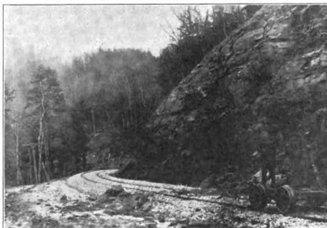
Track and Cut near Elmore, W. Va.; Deepwater Railway.
