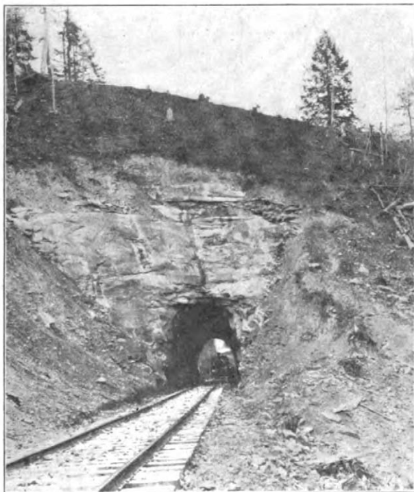
Portal of Tunnel at Mile Post 58; Deepwater Railway.
