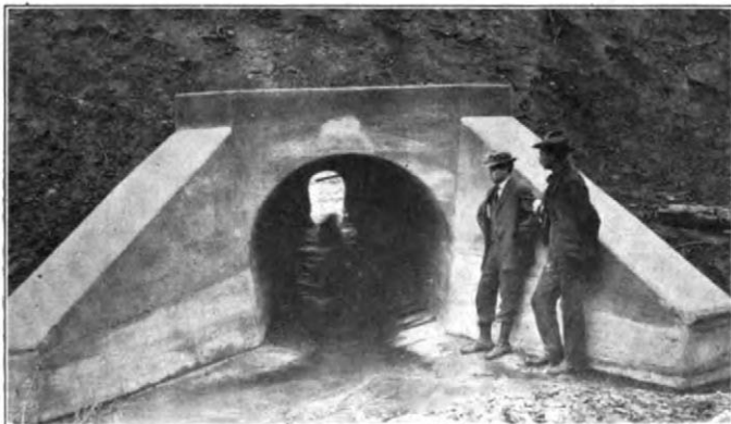
Arch Culvert; Tidewater Railway.
