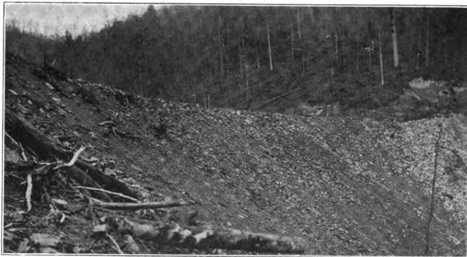
125-ft. Fill at Micajah Gap; Deepwater Railway.
