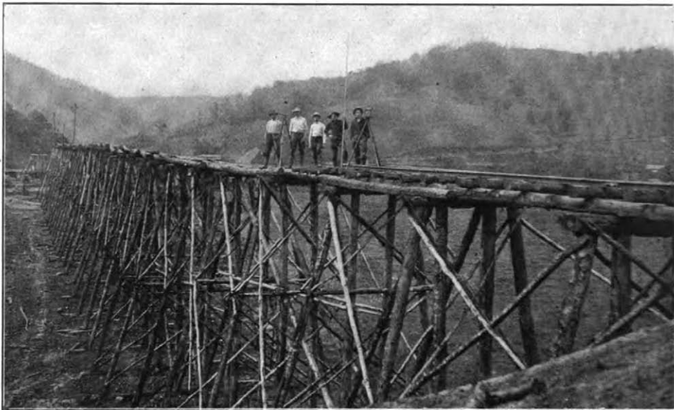
Preparing to Fill at Rock, W. Va.; Deepwater Railway.
