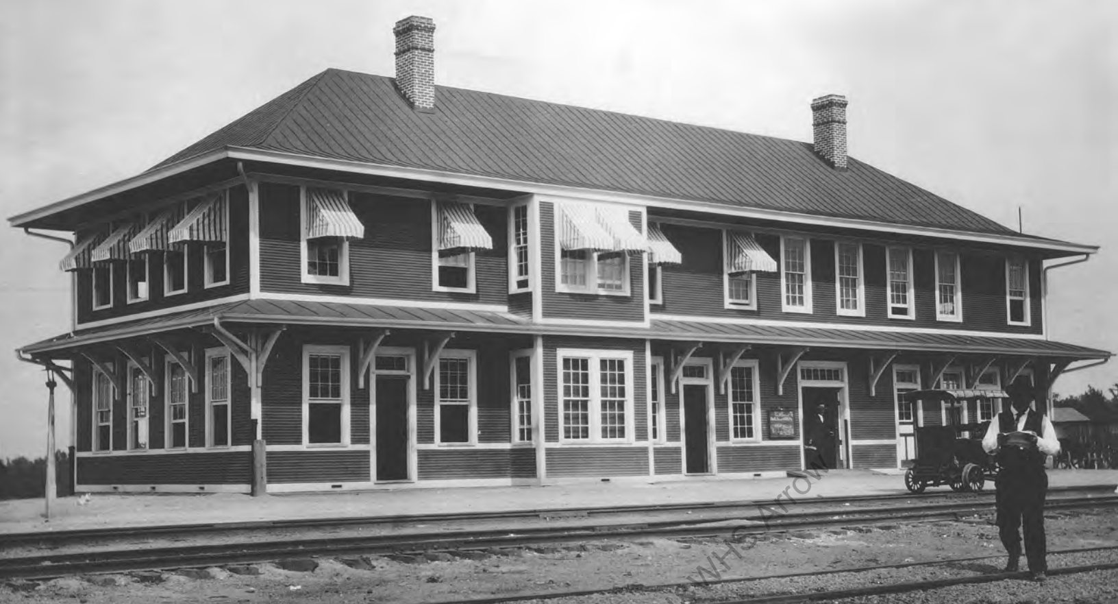
The Virginian's Norfolk division point was Victoria. The station had originally been constructed as a single-story building. In just a few years, the need of a division office brought about adding a second floor. This is obviously fresh paint on August 3, 1910.
