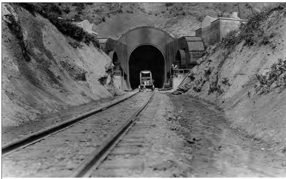
East End, Alleghany Tunnel. M.P. 277.2
