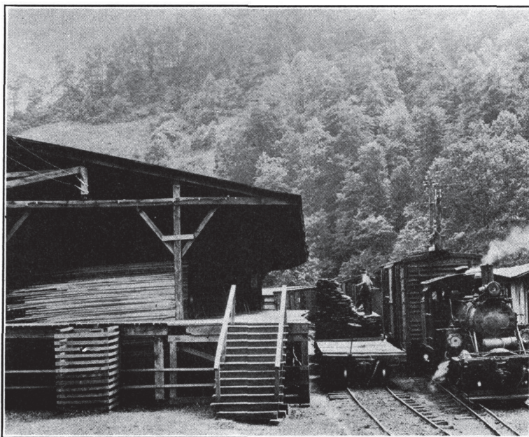
At Lower Elk. Transferring the rough lumber from the narrow gauge flat cars to the standard gauge Norfolk and Western equipment
