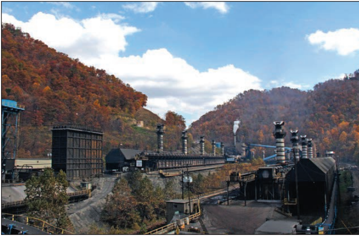
Coal & Coke Plant in Vansant, Virginia Oct 25, 2012
