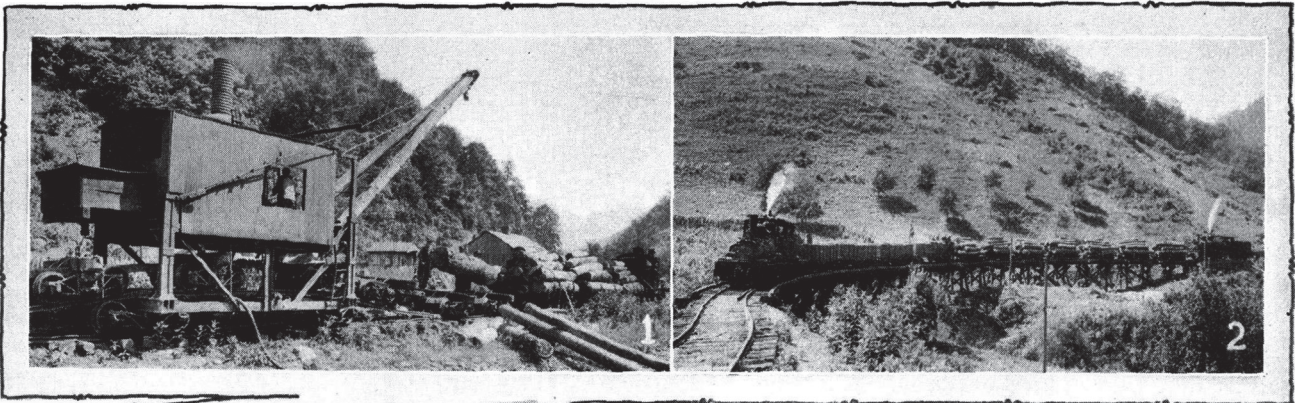
(1) The steam loader at work loading the log cars. (2) A log train pulling a heavy grade near "Rock House Gap," on its way to Blackey. (3) One of the Ritter sawmills, showing the log pond and the "jack slip" which carries the logs from the pond to the mill. (4) Interior of the sawmill at Hurley. Here the boards are shown just after the sawing process, being inspected and graded. The grader is shown at the extreme right examining a board
