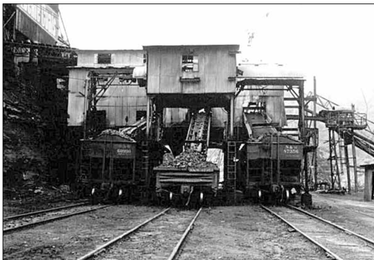
Top to Bottom: Buchanan County Coal Corporation No. 1 (T-96), Buchanan County Coal Corporation No. 2 (T-97), and Panther Coal Company Operation No. 1 (T-100) were photographed in August 1956 and published in the September 1956 Norfolk and Western Magazine .
