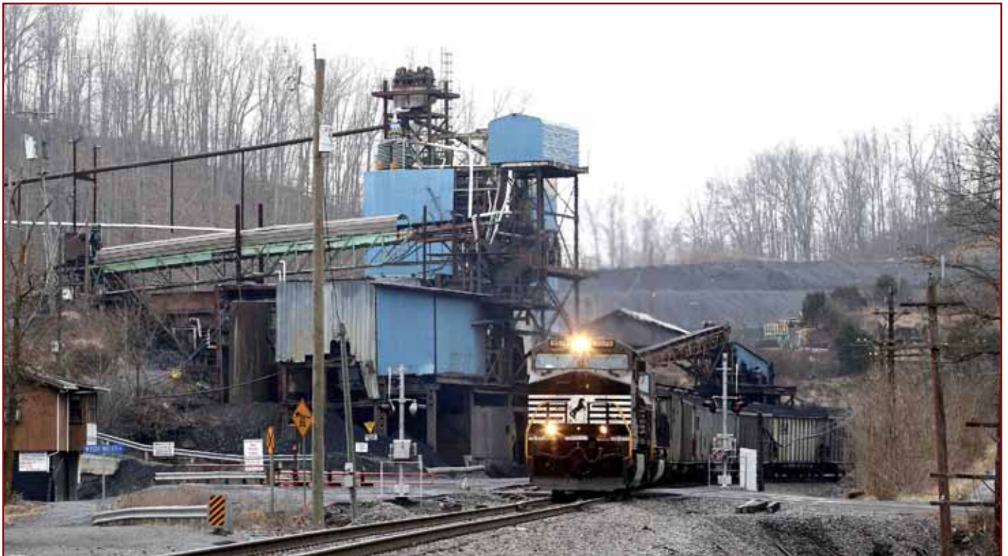
This 2012 photograph shows just part of CONSOL Energy's Buchanan No. 1 mining operation at Oakwood/Page, VA. Constructed in the early 1980s, the mine has a capacity of about 400,000 tons of coal per month. Read about this mine and the other mines on the Buchanan/Levisa/Dismal Creek Branches in the short history of mining on the branches included with this eTAF. Ed Painter photograph
