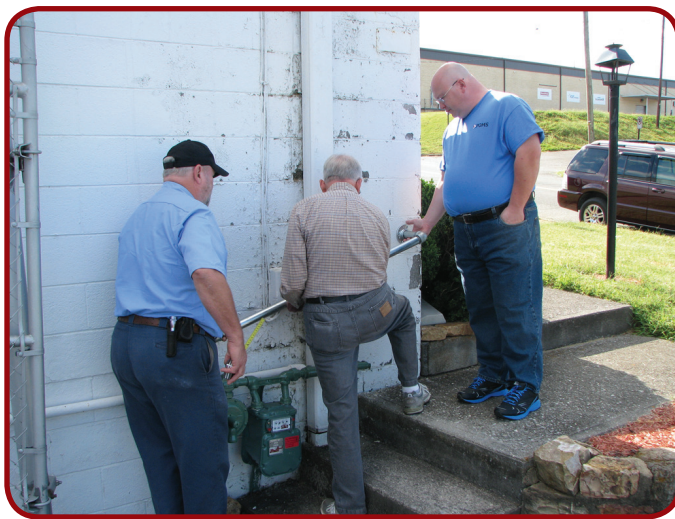
Ben Shank, Gordon Hamilton and Joe Shaw spent part of their time at the September 2013 Archives work session installing a hand-rail for the steps leading into the NWHS building. Alex Schust photo
